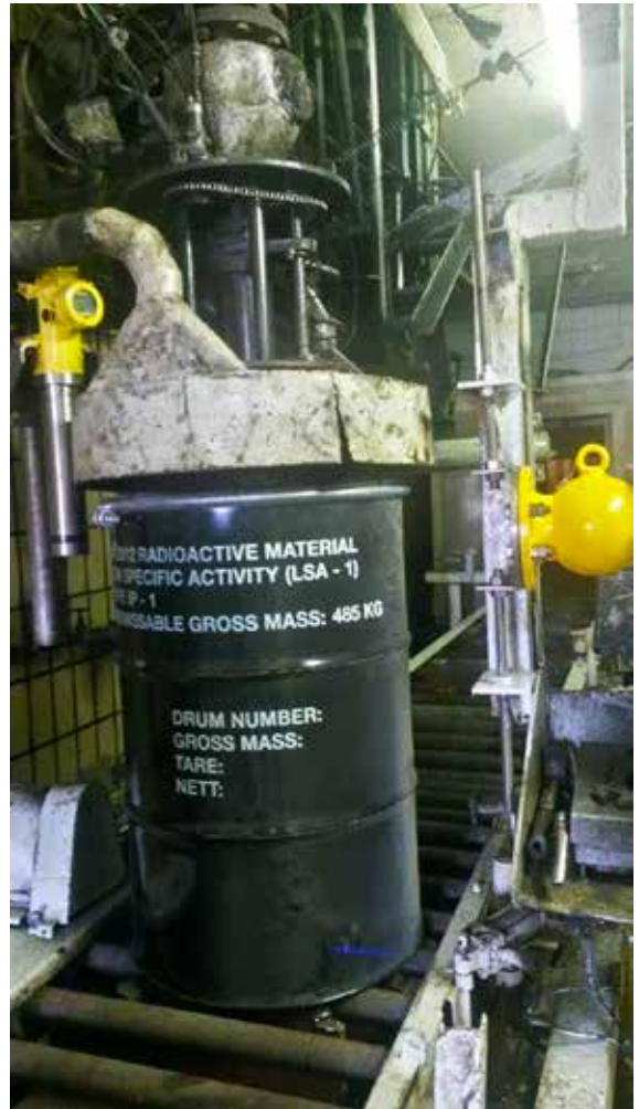
Figure 6: New sealed source for measuring drum filling levels in Final Product Recovery area
